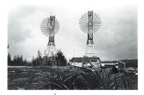
Shown is the 30-foot parabolic aluminum mesh troposcatter antenna system manufactured by Comtech Antenna Systems, Inc. The system provides a data and voice communications link between mainland Malaysia and an off-shore oil platform. The electronics for this system was provided jointly by Comtech Microwave Corp. and Comtech Systems, Inc.
