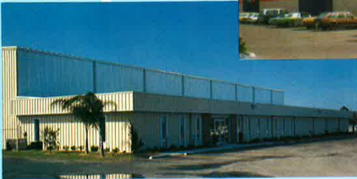
COMTECH ANTENNA CORP. St. Cloud, Florida
