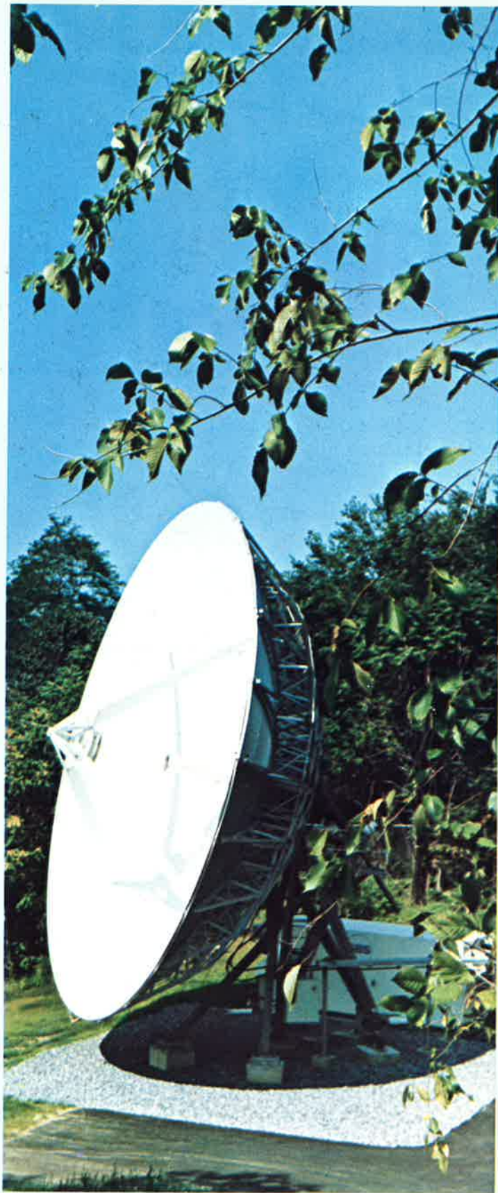
Two data-only earth stations, manufactured and installed by Comtech for Satellite Business Systems Inc., provide a satellite communications data link between the east (Poughkeepsie, N.Y.) and west coasts (Los Gatos, California). Currently, this satellite link is undergoing development tests for direct high-speed digital, and time-division multiple-access (TDMA) transmissions via an existing geostationary domestic satellite. The earth stations contain Comtech's highly-reliable C-band communication equipment and antennas. An additional earth station, currently being manufactured by Comtech, will be located at the Research Triangle Park site in Raleigh, North Carolina.
