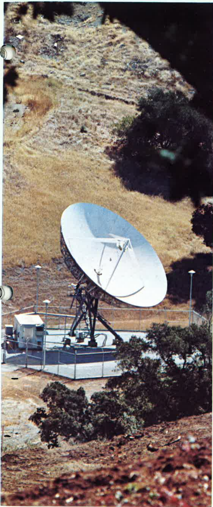
Two data-only earth stations, manufactured and installed by Comtech for Satellite Business Systems Inc., provide a satellite communications data link between the east (Poughkeepsie, N.Y.) and west coasts (Los Gatos, California). Currently, this satellite link is undergoing development tests for direct high-speed digital, and time-division multiple-access (TDMA) transmissions via an existing geostationary domestic satellite. The earth stations contain Comtech's highly-reliable C-band communication equipment and antennas. An additional earth station, currently being manufactured by Comtech, will be located at the Research Triangle Park site in Raleigh, North Carolina.
