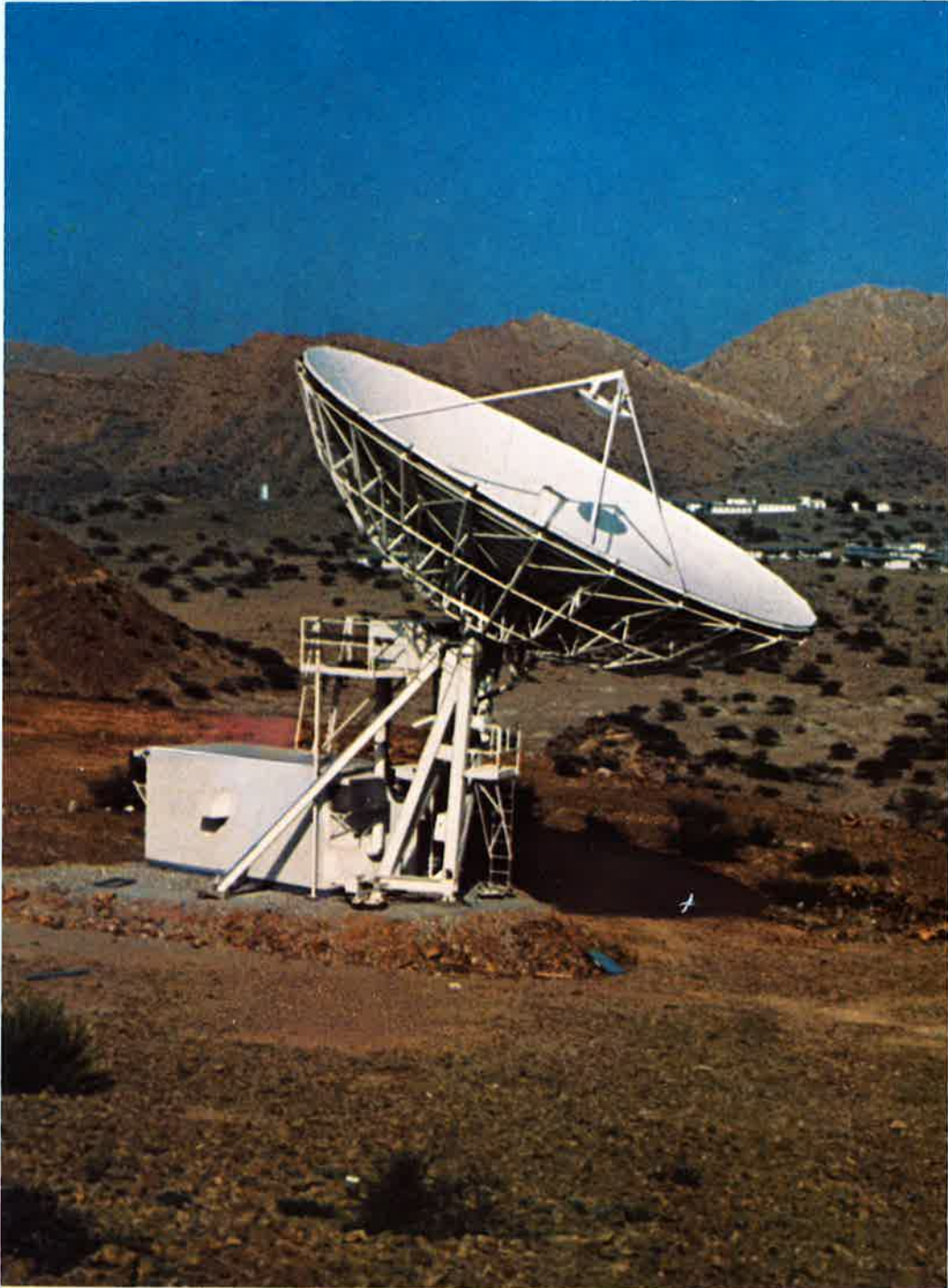
Medium-Size Intelsat Earth Station Installed By Comtech In Oman For Cable And Wireless Ltd.
